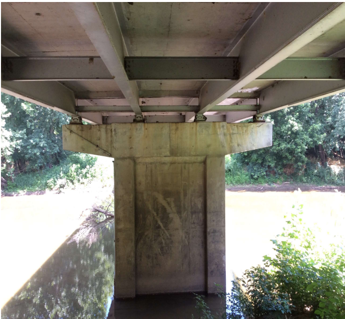
PHOTO 1 Description Span # 1 Bent # 2 horizontal cracking in cap.
