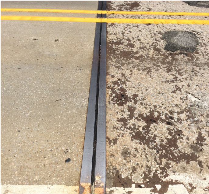
PHOTO 1 Description Bent # 2 failing joint seal.
