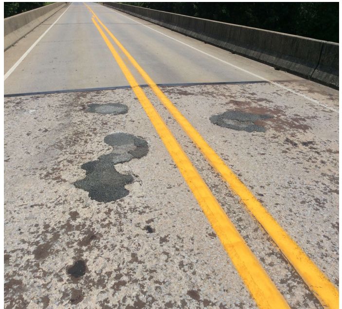
PHOTO 2 Description Span # 1 temporary asphalt repairs.
