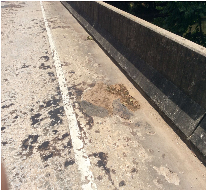
PHOTO 1 Description Span # 1 Right gutter pothole.
